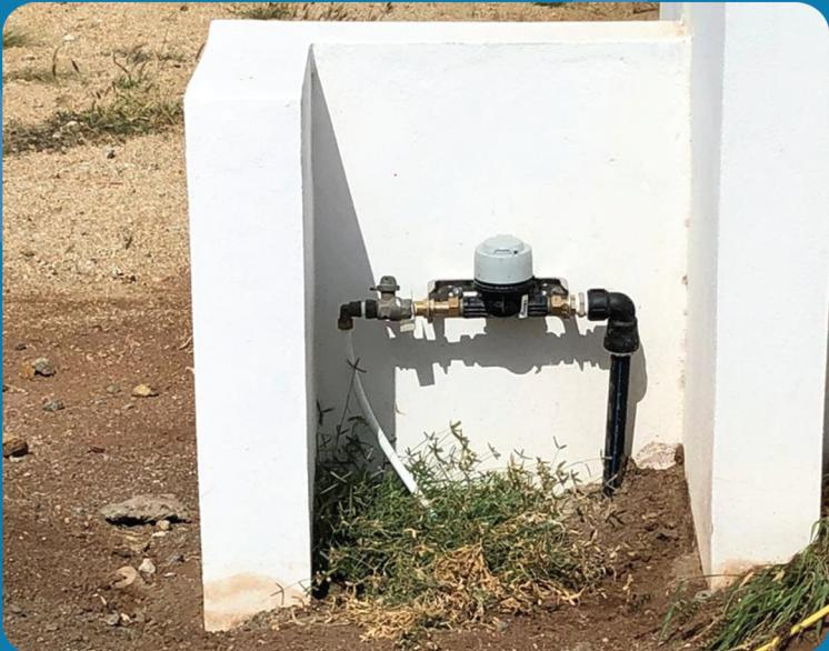
\*: A 'niche' is a concrete enclosure that is open in the front and on the top and closed on both sides.
